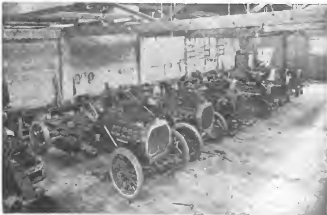
GEARLESS CARS IN PROCESS OF CONSTRUCTION.
